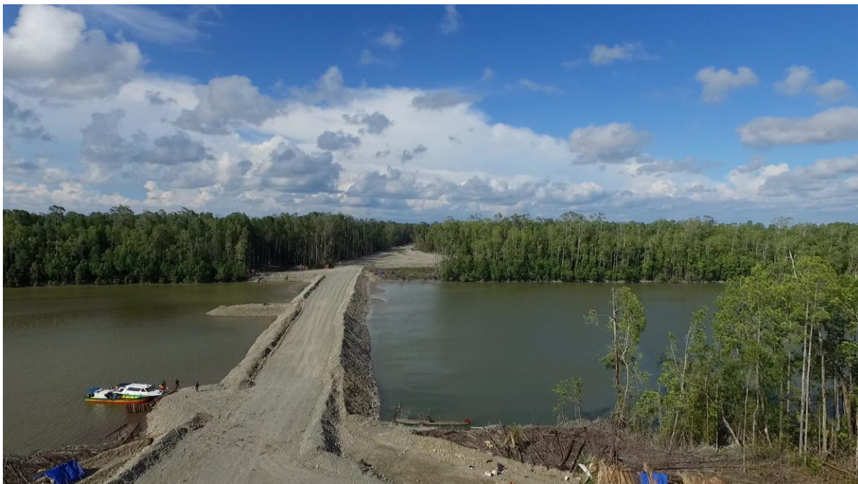
Yamaima River cut off by dyke, so that tailings slurry sediment does not cause siltation at Freeport's port. Right side flows from tailings deposition, left side flows to the sea.
