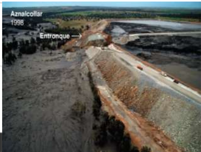
Fig 5: Collapse of Aznalcollar dam (1998)
